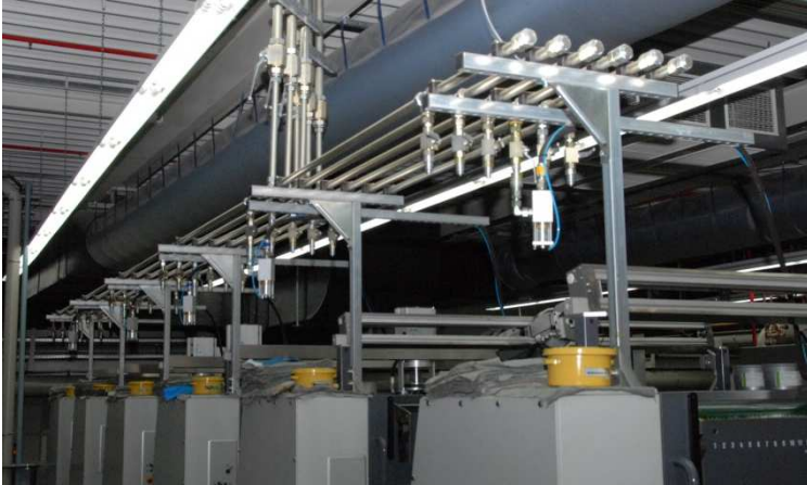
BCP with ABB-control station connection
